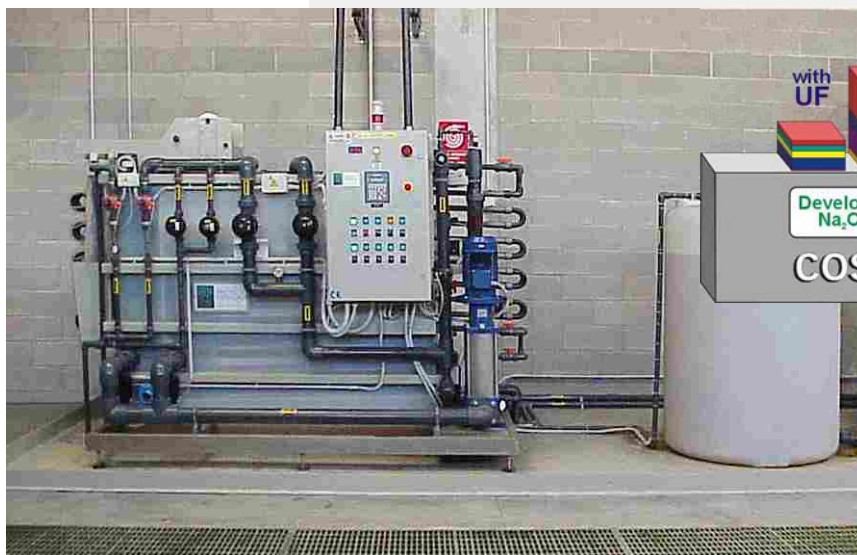
UF STRIP unit - mod. 10TA - with permeate storage tank
